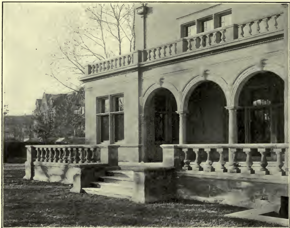
FIG. 13.—SOUTH PORCH OF THE SCHLESINGER HOUSE.
